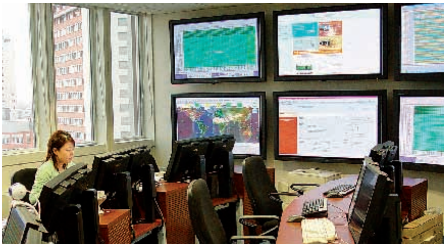
Control room of the Operations Centre.
