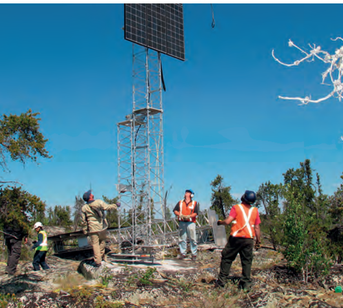
Upgrading work at primary seismic array station PS9, Yellowknife, Northwest Territories, Canada. Left: Erection of solar panels. Right: Installation of an equipment enclosure.
