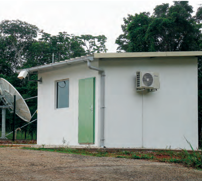
Auxiliary seismic station AS33, Montagne des Pères, French Guiana, which was certified in 2012.
