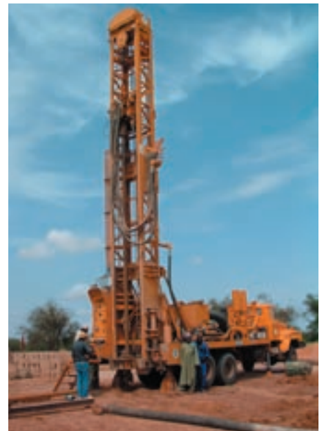
DRILLING OF BOREHOLES AT PS26, TORODI, NIGER, APRIL 2005
