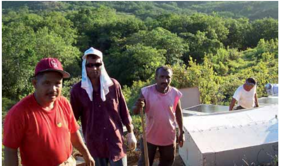
PALAUAN WORKERS CONSTRUCTING THE REPEATER SITE OF INFRASOUND STATION IS39, PALAU
