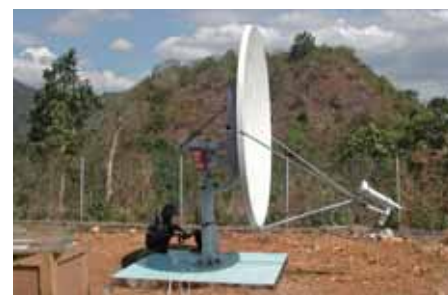
INSTALLATION OF GCI ANTENNA, AS44, KAPPANG, INDONESIA, NOVEMBER 2002
