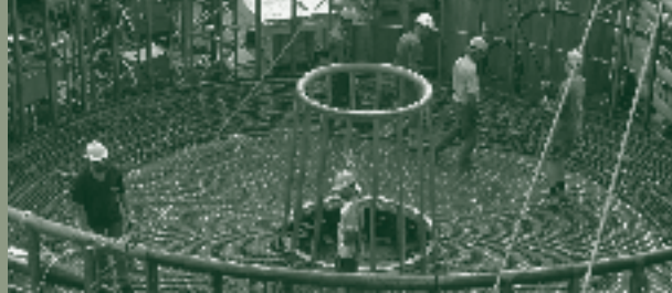
LAYING THE CABLES FOR HYDROACOUSTIC STATION (HA05) IN MARTINIQUE, FRANCE
