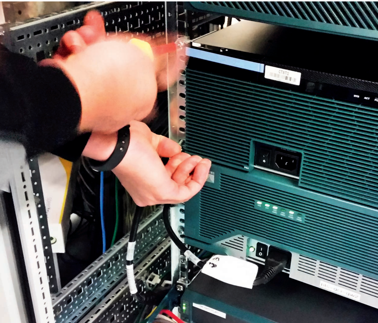
Installation of new GCI equipment at the computer centre in Vienna.
