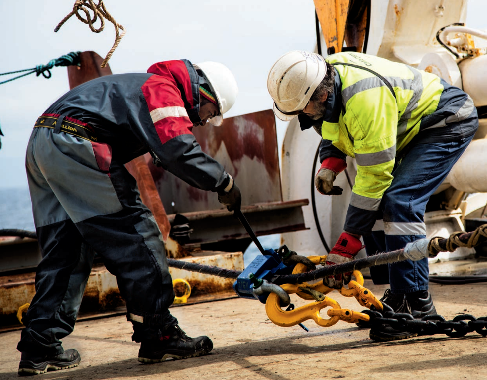
Installation of hydroacoustic station HA4, Crozet Islands (France).
