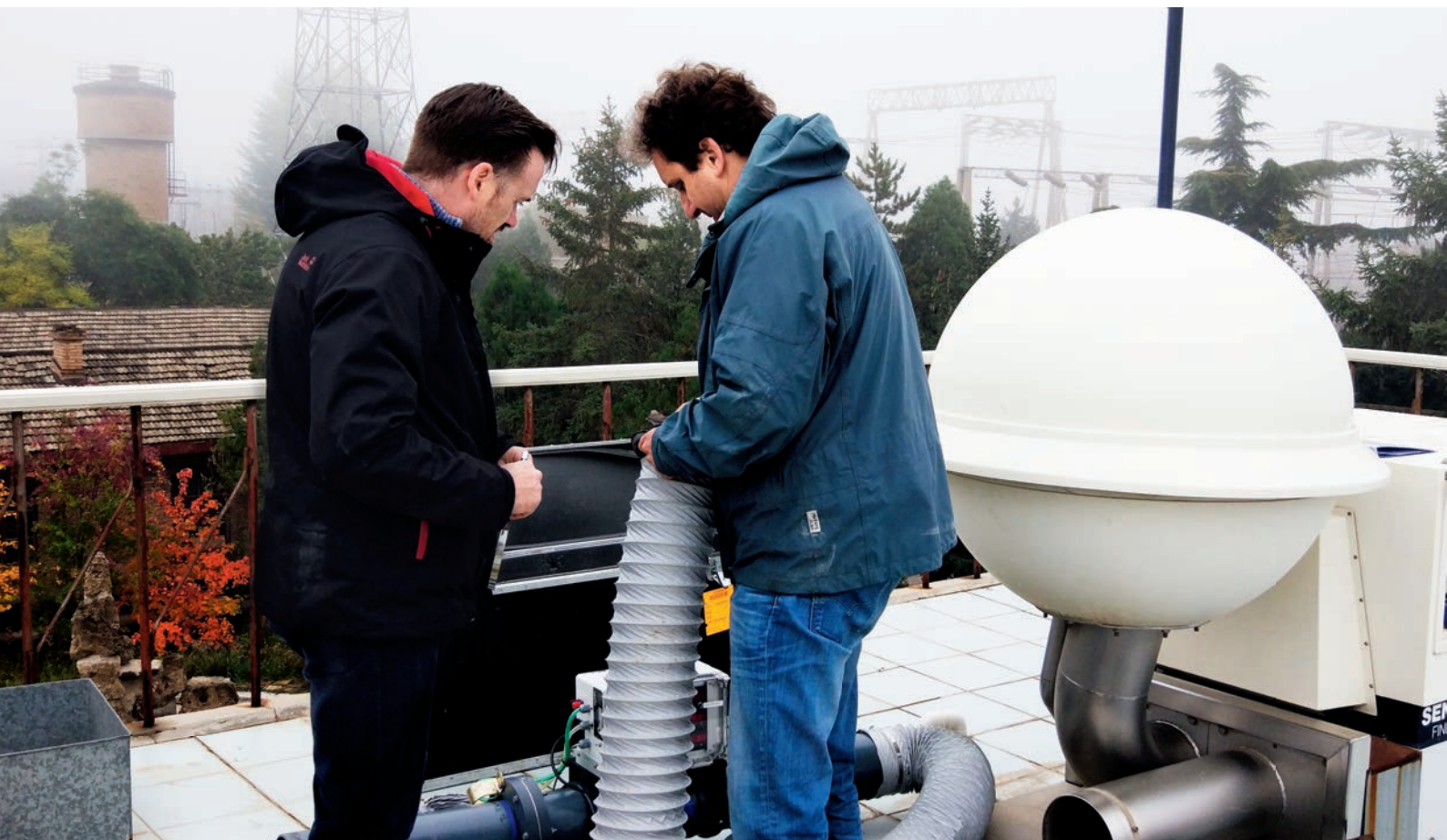
Installation of radionuclide station RN21, Lanzhou (China).
