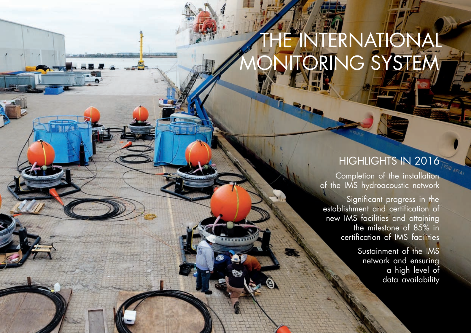
Installation of hydroacoustic station HA4, Crozet Islands (France).
