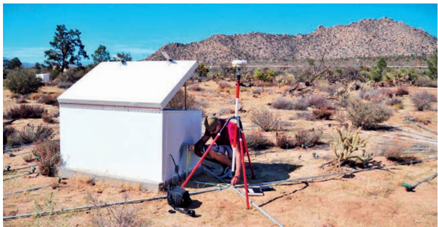
Infrasound station IS57, Piñon Flat, California (USA).
