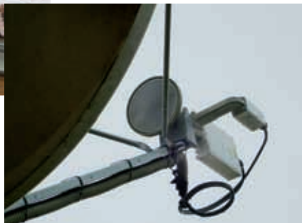
VSAT antenna at PS40, Sonseca, Spain: a clear line of sight to a geosynchronous satellite is the first prerequisite for a VSAT to be able to function as part of the global communications network.
